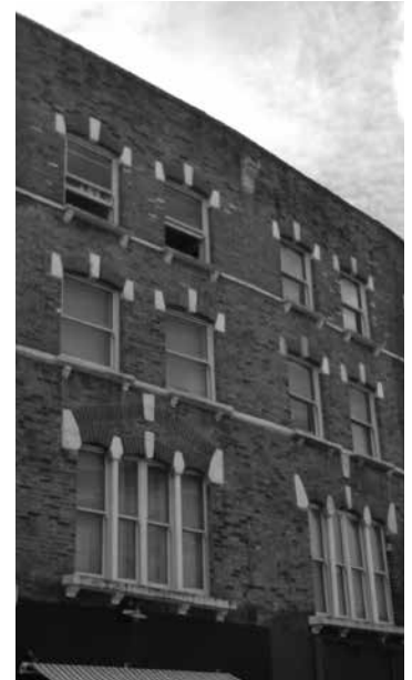
Renovated flats on Camden High Street
